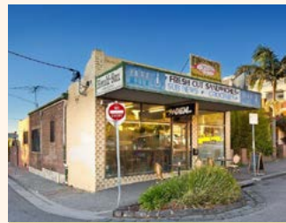
163 Lennox Street RICHMOND. $1,110,000. Mixed use. Development site for 2 - 3 townhouses.
