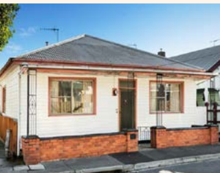
86 Neptune Street Richmond. Sold for $876,000. Corner site with potential for 2 x townhouses.
