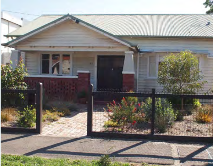
TYPICAL EXAMPLE OF THE BUNGALOW STYLE
