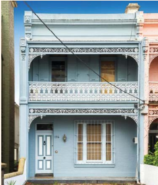
136 Powlett Street East Melbourne
