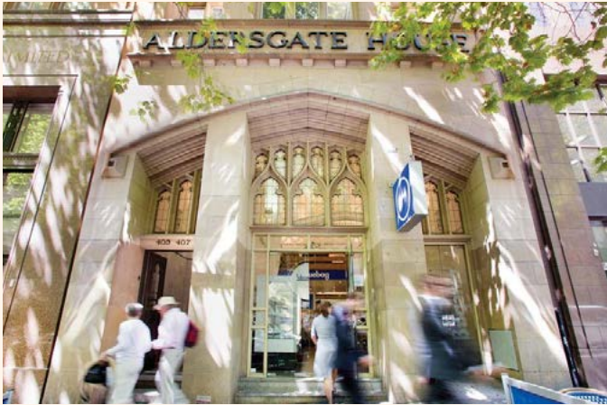
L2 405 Collins Street, Melbourne
